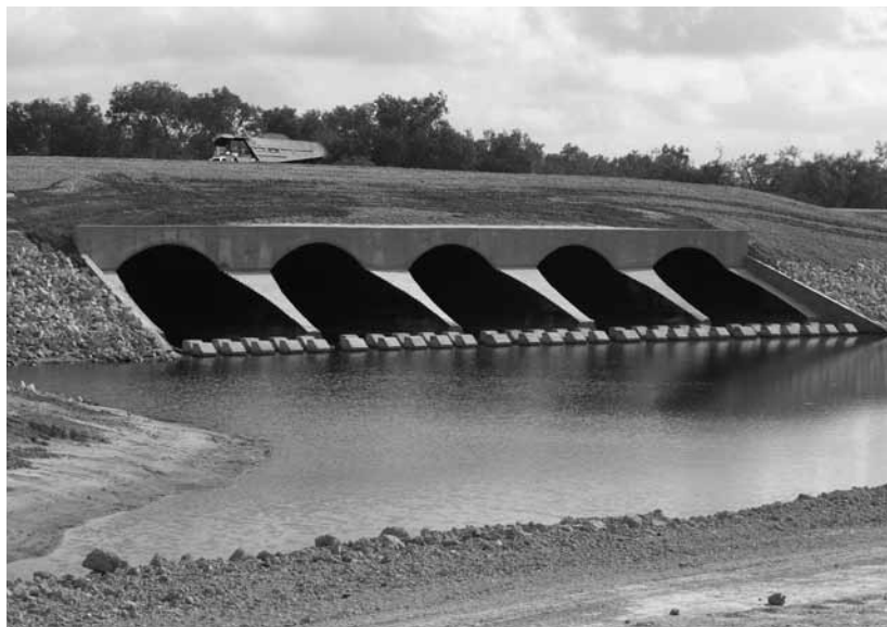
Figure 13. Multiple Barrel Installation with Step-Beveled End Treatment.
