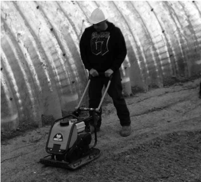
Figure 28. Adequate, uniform compaction is critical to building soil/steel structures.
