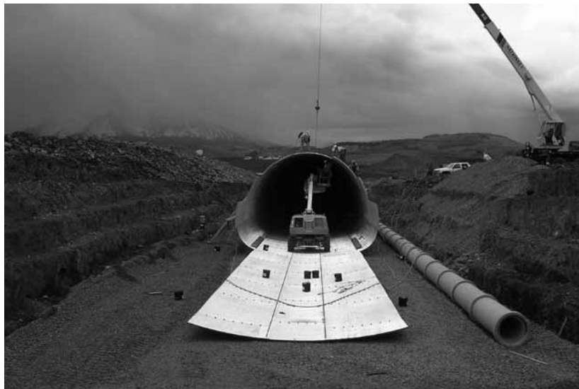
Figure 12 Modern erection techniques are used in assembling structural plate.
