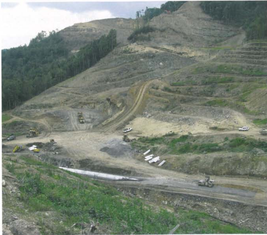
Filling a ravine was necessary to create the new road.
