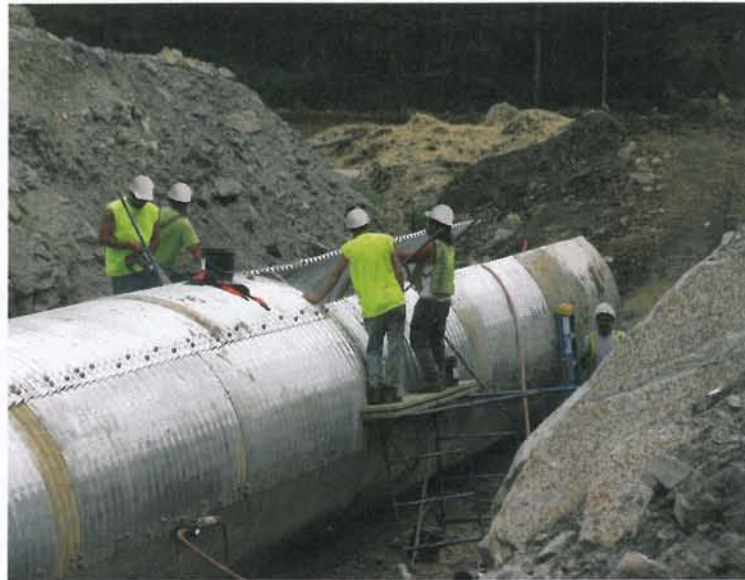
The curved steel plates—490 in all—were assembled and bolted onsite.
