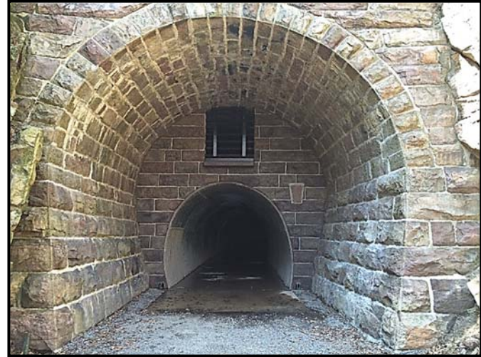
Renovation of the Poe Paddy Tunnel highlights the cooperative venture of State agencies, commissions and associations to meet the safety needs of the public while preserving and protecting a unique aspect of its environment.
