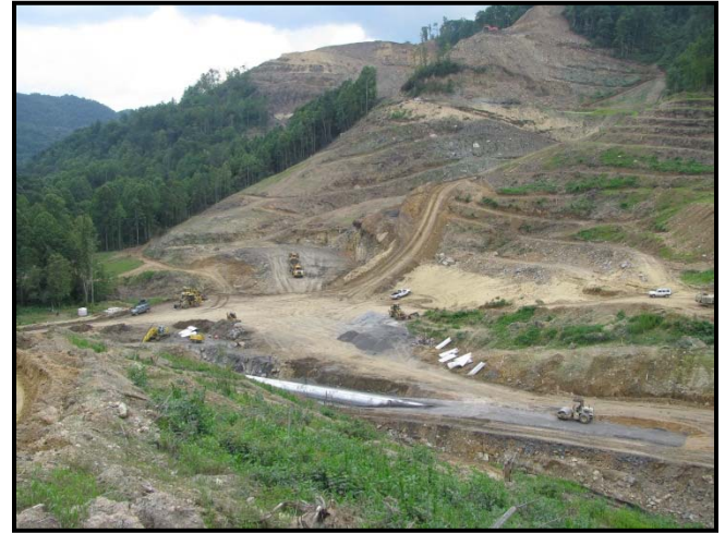
Wyco Hollow at the headwaters of Allen Creek. Vantage point at final grade of the ravine crossing. An estimated three million cubic yards of fill needed to reach grade opposite side (notch to the right of upper middle tree line).
