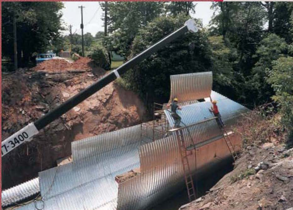
Structural Plate Pipe 22 feet in diameter, Elongated Railroad Tunnel
