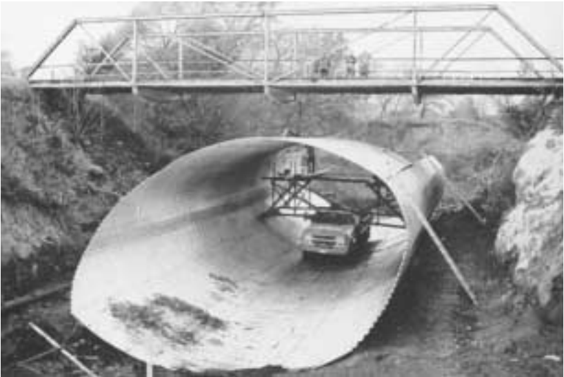
Figure 7. Modern erection techniques are used in assembling structural plate.
