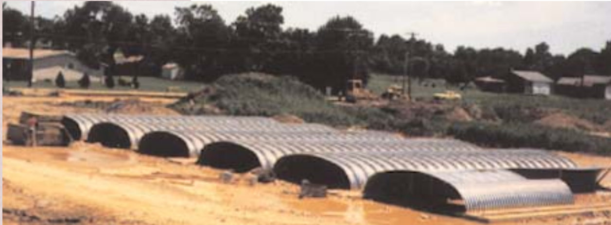
Box culvert at residential development entrance.
