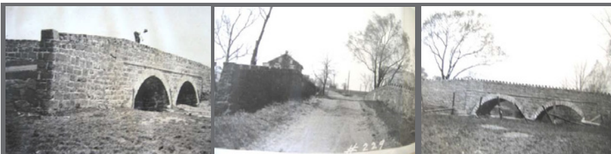
Earliest photos of record taken during a 1916 inspection of the Eleventh Street Bridge (photos courtesy of Montgomery County Department of Roads and Bridges).
