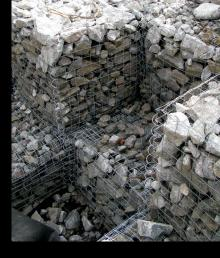
Lane gabions and mattresses meet ASTM A974 in regard to the material used and the method of manufacture. ASTM A974 also establishes minimum requirements for preassembly of the baskets and mattresses for shipping. The wire mesh used is galvanized or PVC coated. PVC-coated gabions are used in applications where greater durability or an environmentally-blended appearance is desired.
